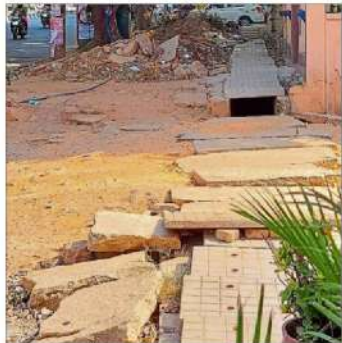
This footpath near the KFC and Pai International signal in Indiranagar was dug up about six months ago and is still not fixed.
