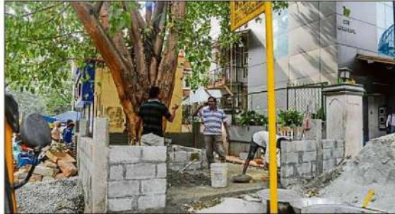
The construction of the 'arali katte' at Jogupalya ward No 89, Indiranagar. DH PHOTO/S K DINESH
