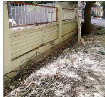
Dry leaves falling on the roadside clog the stormwater drains at 23rd Main, HSR Layout Sector 1.
