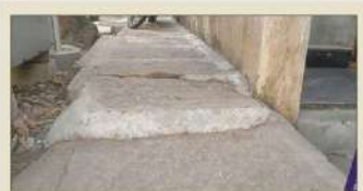
The footpath at the junction of 5th Main and 6th Cross Malleswaram was repaired in a hurry. And the shoddy work is there for all to see.
