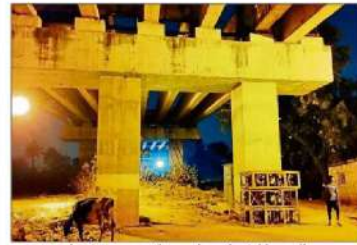
Nearly 10 years on, the work on the Jakkur railway flyover is still incomplete.
